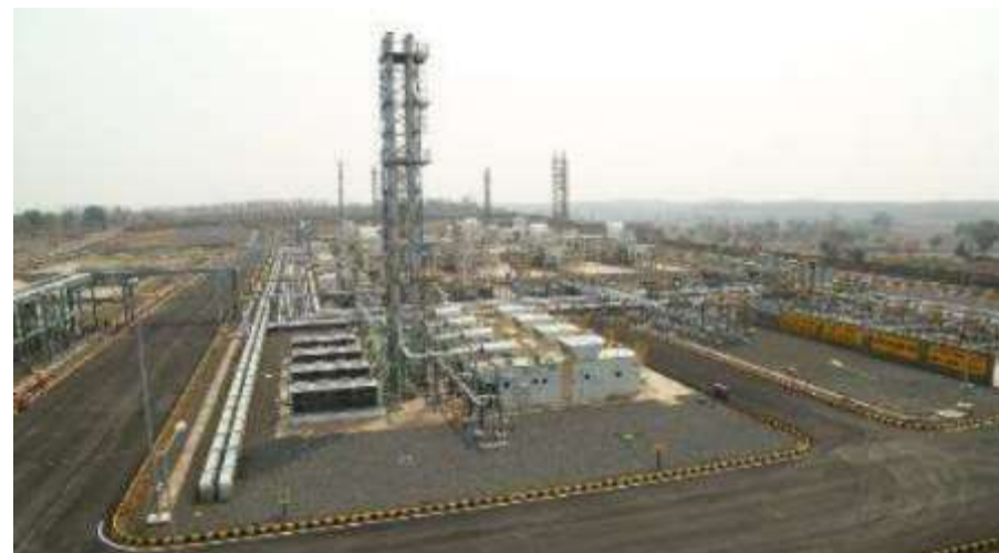
Installation of GGS-11 completed
