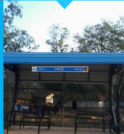
Metal Beam Crash Barrier
