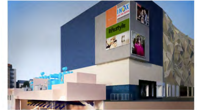
Underground 132 kV SS at 'Quest Mall'
