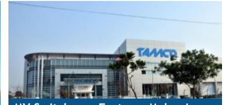
MV Switchgear Factory, Malaysia
