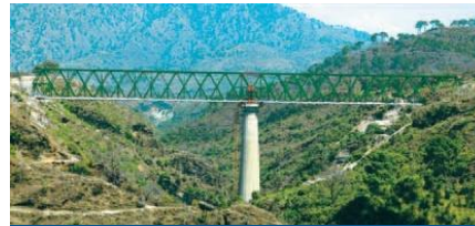
88m Rail Bridge Jammu Udhampur
