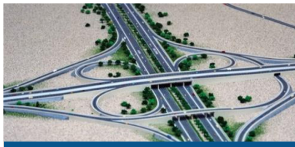
Sheikh Khalifa Interchange, UAE
