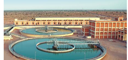
Water Treatment Plant, Barmer
