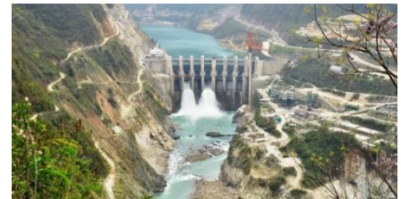
Srinagar Hydro Electric Plant
