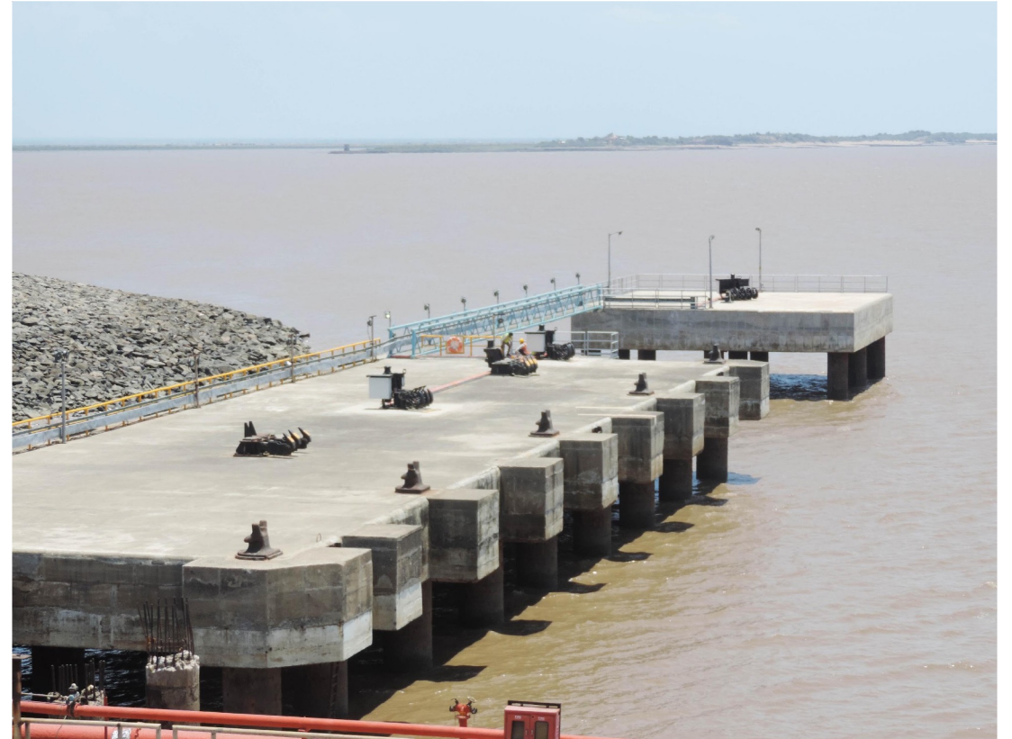
Pipavav Jetty infrastructure upgrade
