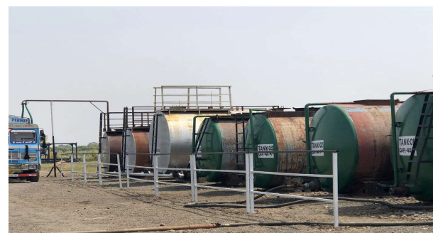
Jyoti I – Oil Storage
