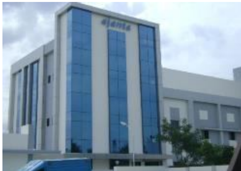
API Plant - Waluj
