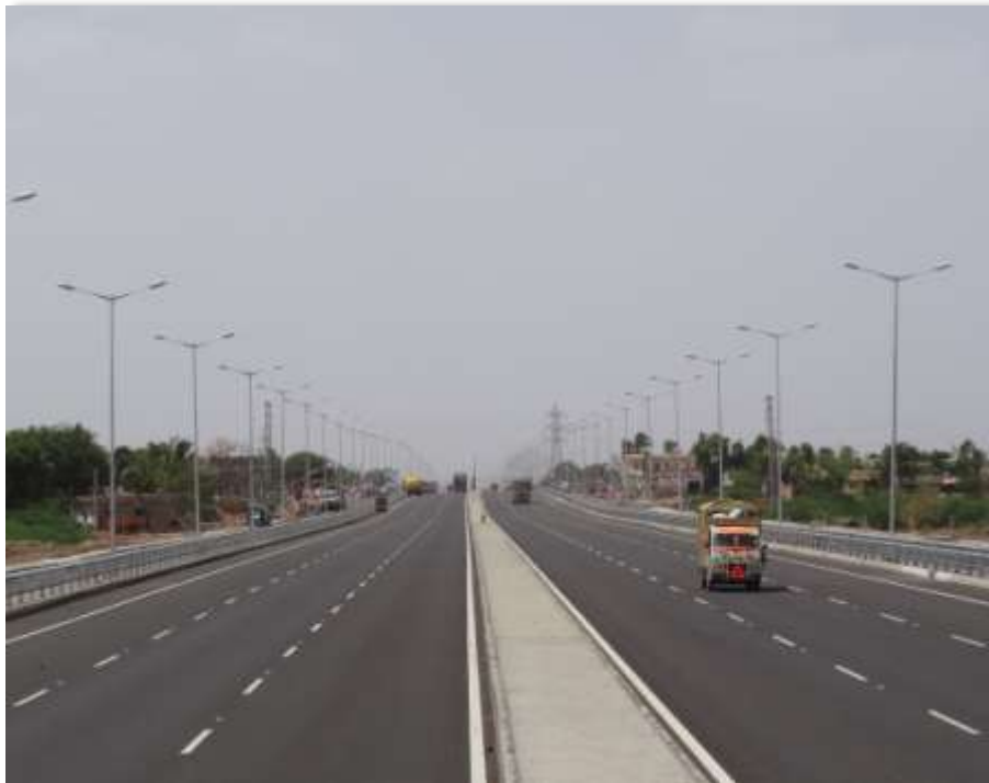
Road Project in the state of Karnataka - Bijapur - Hungund
