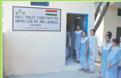
Toilets constructed in schools in Nangal
