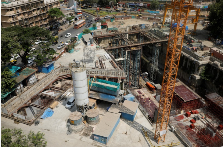
Piling at Mumbai Underground Metro Project
