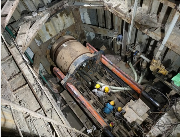
Micro Tunnelling Project, Kolkata
