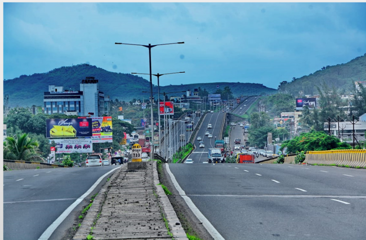
Pune Satara Road Project
