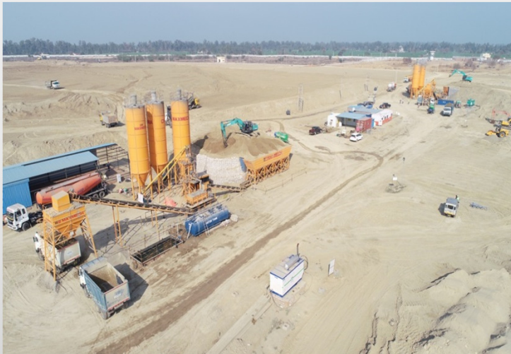
Ground Stabilisation work for Nuclear Power Corporation
