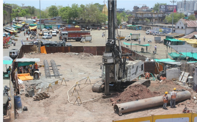
Piling Work at Nagpur Metro
