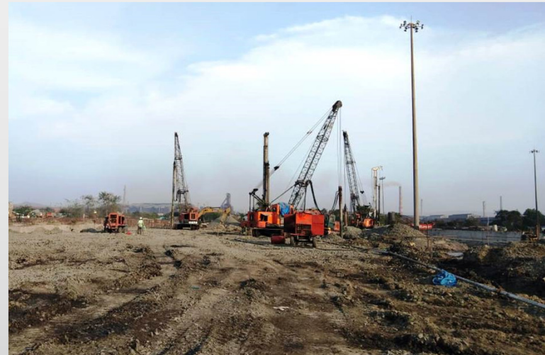
Stone Column Work at Jindal Steel
