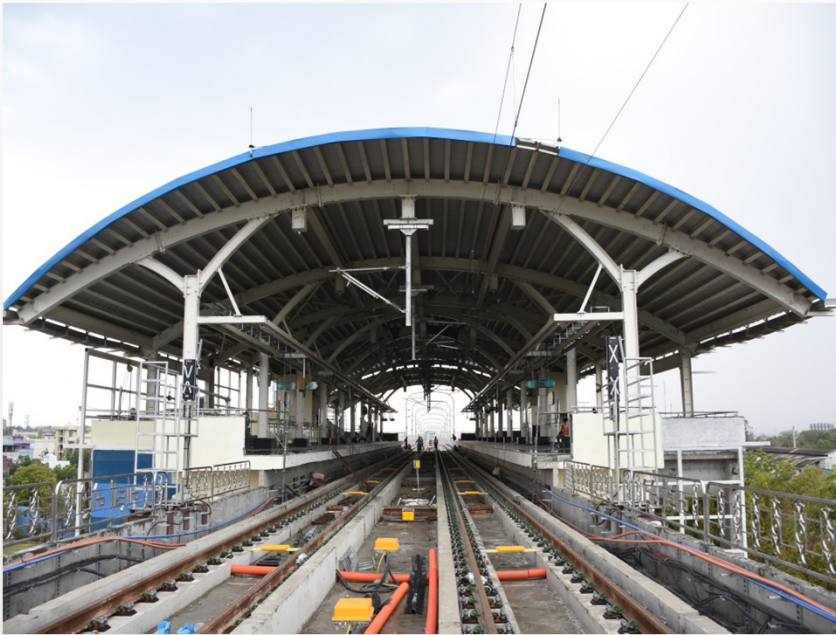
Nagpur Metro Project
