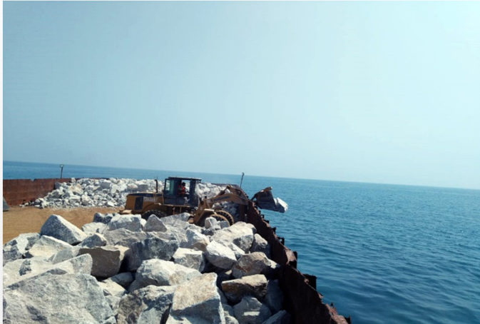
Rock Placing, Udangudi Project
