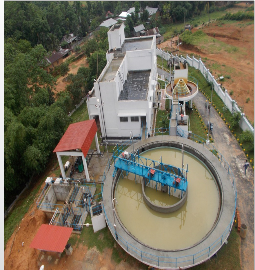
Agartala WTP project
