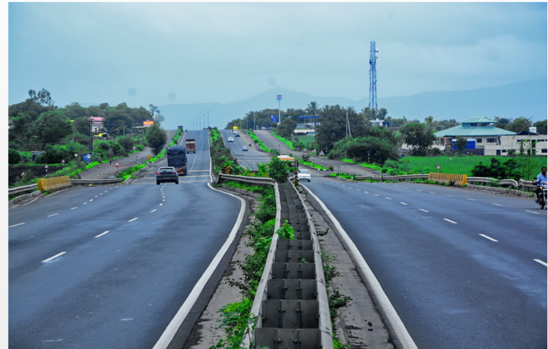
Pune Satara Road Project
