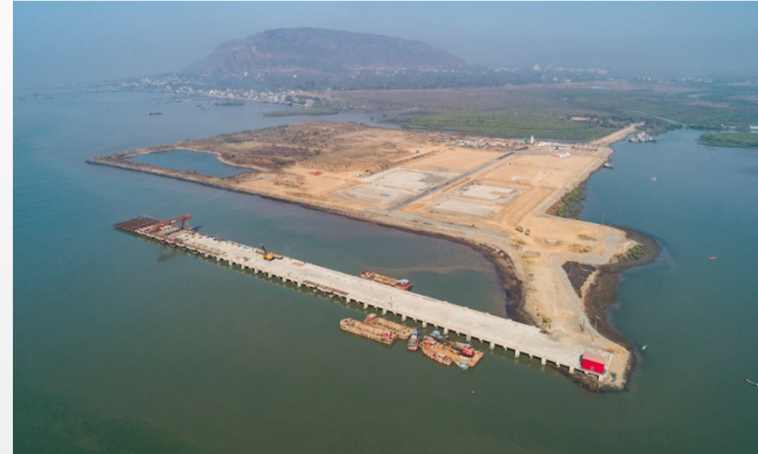
Karanja Port Project
