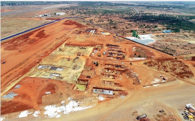
Trichy Airport Modernisation
