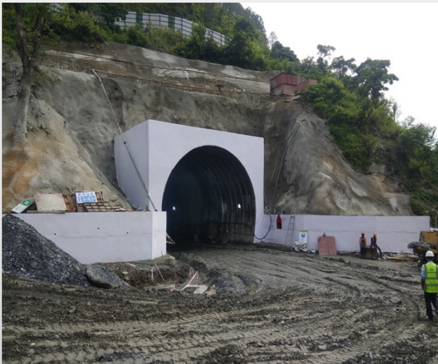
Tunnel for Indian Railways, Uttarakhand
