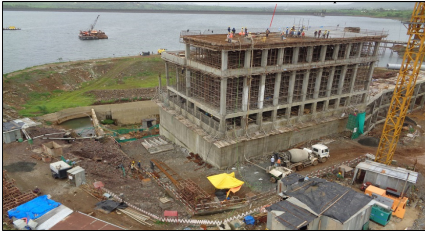
Bhama Ashed Water Supply Project
