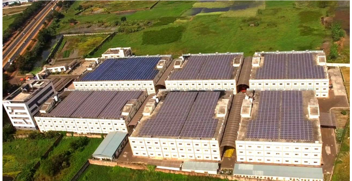
Rooftop solar power plant at Dankuni unit
