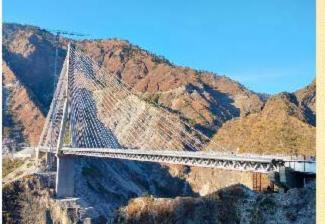
Anji Khad Bridge: Most of the Civil work is over and finishing works such as slope stabilization, Aerodynamic structure, Crash barrier works are in progress.
