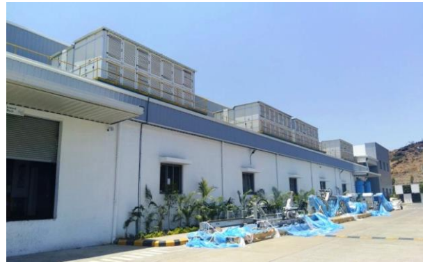
Kalyani Technoforge Ltd – Pune
