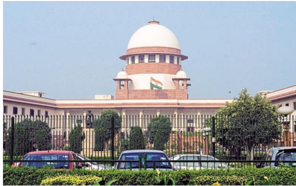
Supreme Court, Delhi (Extension project) Boards for ceilings & windows
