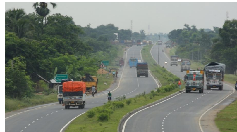
Km 341 (Farakka Raiganj Highway)
