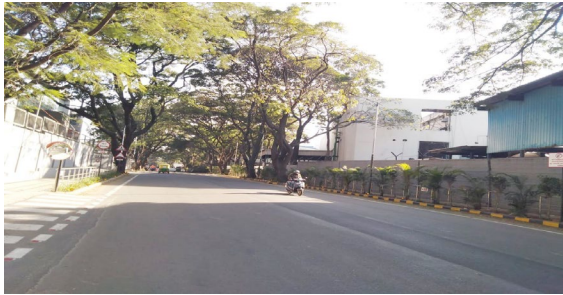
Peenya Public road and infrastructure upgradation near 80% completion with ABB circle
