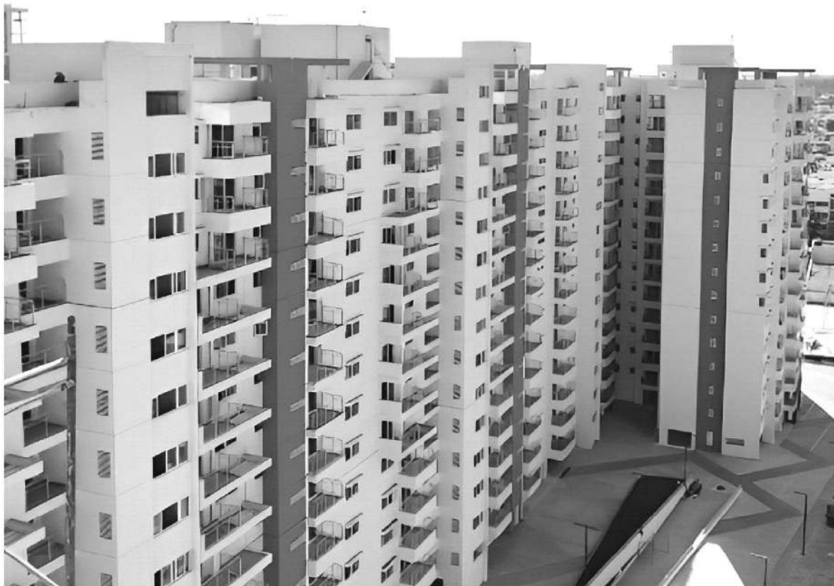
Sattva Navaratna Residency Apartments for M/s Sattva Group at Coimbatore, Tamil Nadu.
