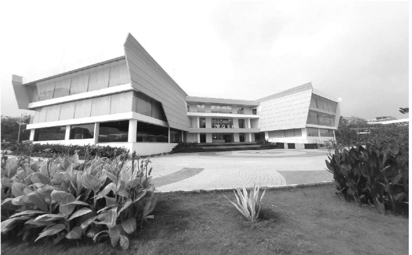
(Welcome Group School of Hotel Administration – WGSHA ) Academic block building for M/s Manipal Academy of Higher Education at Manipal, Karnataka.
