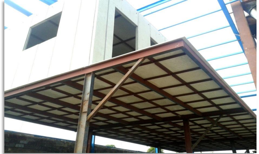
Mezzanine flooring - (V-Board)
