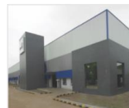
Foundry Division, Vambori
