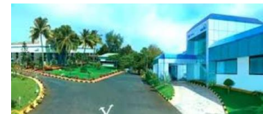
KSB MIL Controls Ltd. Meladoor, Kerela
