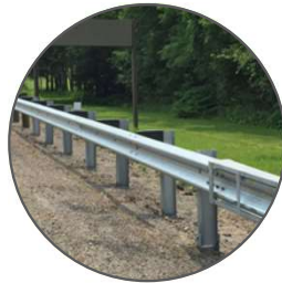
Metal Beam Crash Barrier
