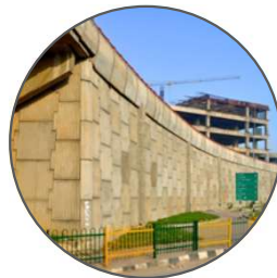
Reinforced Earth Walls
