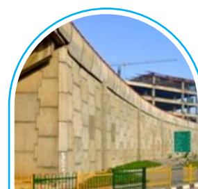
Reinforced Earth Walls
