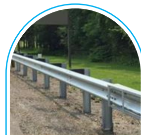
Metal Beam Crash Barrier
