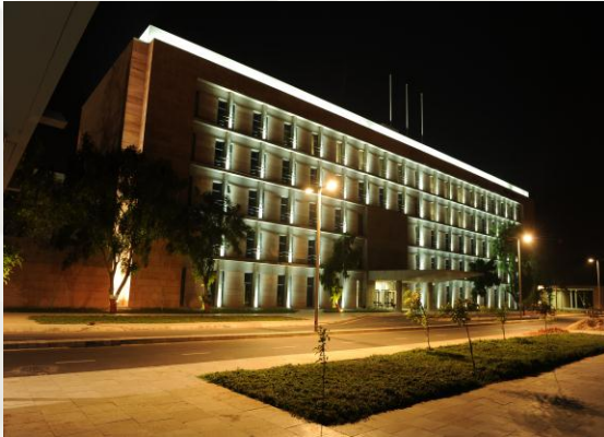
Swarnim Sankul 1 & 2 Construction and interior work
