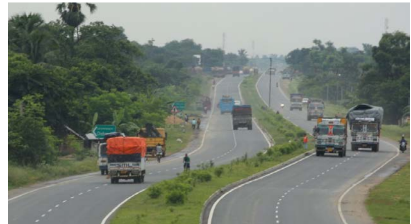
Km 341 (Farakka Raiganj Highway)
