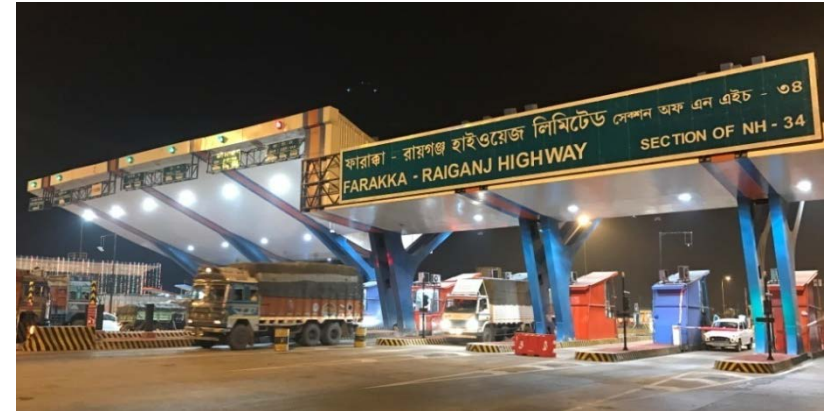
Farakka Raiganj Highway: Toll Plaza at Km 297
