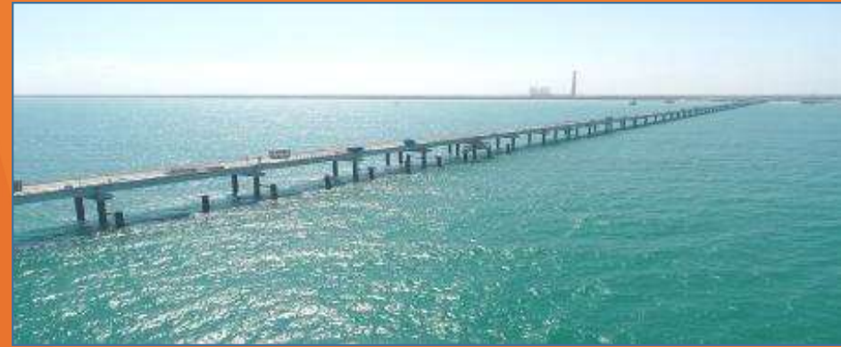
Udangudi Super critical thermal power project in Tamil Nadu
