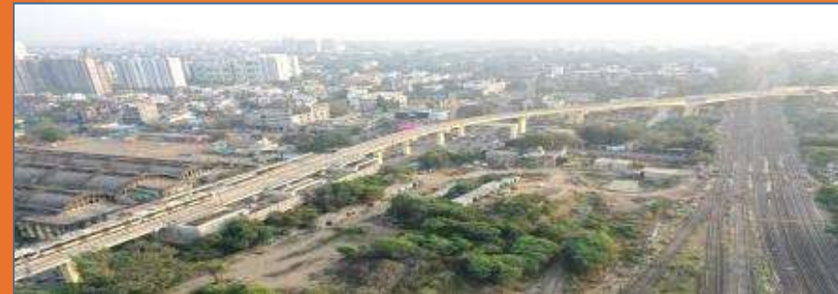
Nagpur Maha Metro cantilever bridge in Maharashtra
