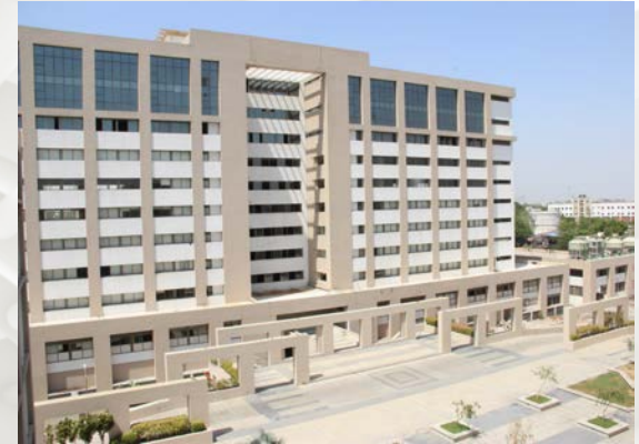
Hospital, Residential Building and Medical College for GCS Medical College, Hospital and Research Centre
