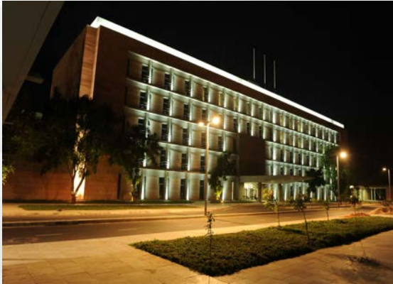
Swarnim Sankul 1 & 2 Construction and interior work
