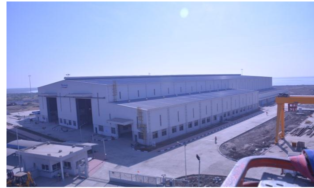
Technip – Dahej, Gujarat
