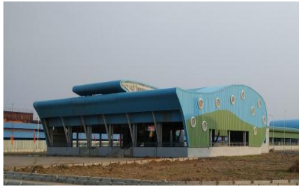
RO-RO Ferry Terminal – Dahej, Gujarat
