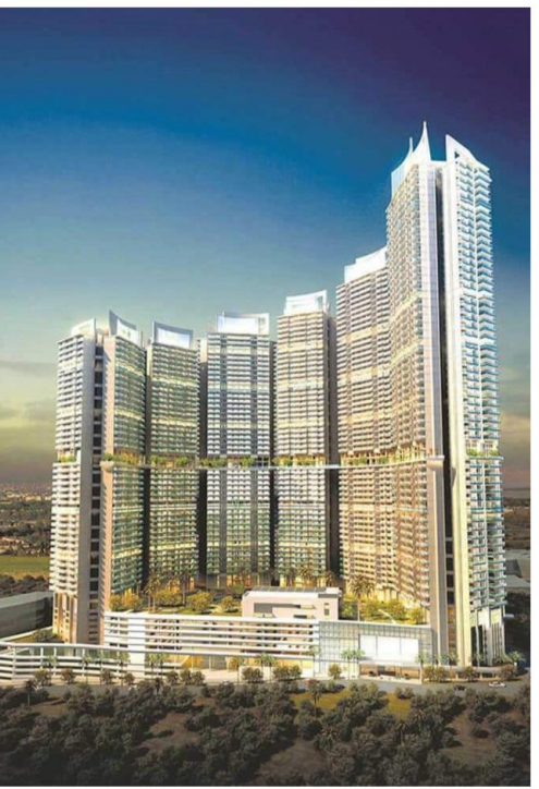
L&T Crescent Bay
