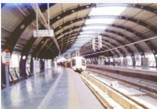
Elevated Metro Stations, DMRC, Delhi
