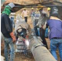
Thumbli Water Pipeline– Cairn Energy India – Rajasthan
