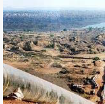
Mundra Bathinda Pipeline Project – HPCL Mittal Pipeline Ltd – Gujarat & Rajasthan
