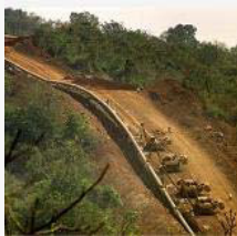
Panvel Dabhol Pipeline Project–Gail Ltd - Maharashtra
