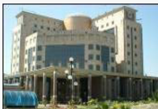
Power Grid Corpn., Gurgaon
