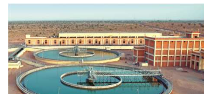
Water Treatment Plant, Barmer
