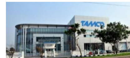
MV Switchgear Factory, Malaysia
