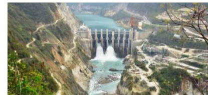
Srinagar Hydro Electric Plant
