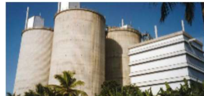
Bulk Cement Terminal, Colombo
