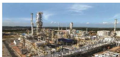
Petronas Refinery, Malaysia
