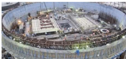
Kakrapar Nuclear Power Plant, Guj
