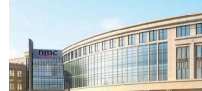
NMC Speciality hospital, Abu Dhabi
