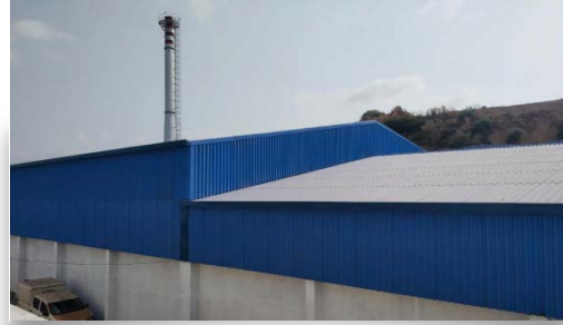
Everest Hi-Tech Yeshaswi Fish & Mill Oil Company, Mangalore
