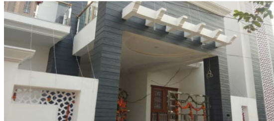
Cladding Residential Site, Bareilly
