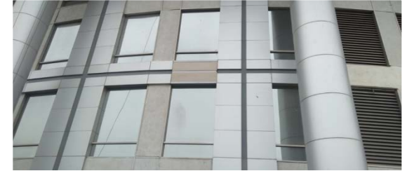
Fibre Cement Boards DLF Cyber city, Gurgaon
