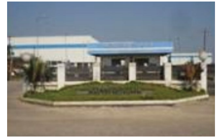
Unit 2 - Chakan, Pune, Maharashtra (Area - 58,364 sqm)
