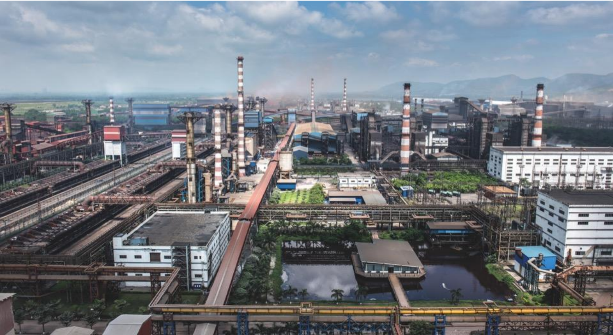
Aerial View of Raigarh Plant
