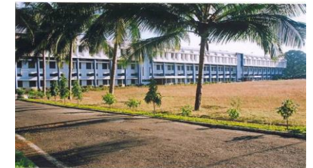
Plant 3 Sirsi, Uttara Kannada Dist., Karnataka
