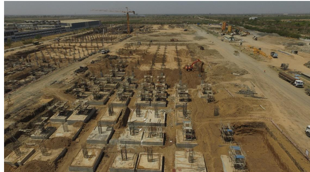
Civil work in progress
