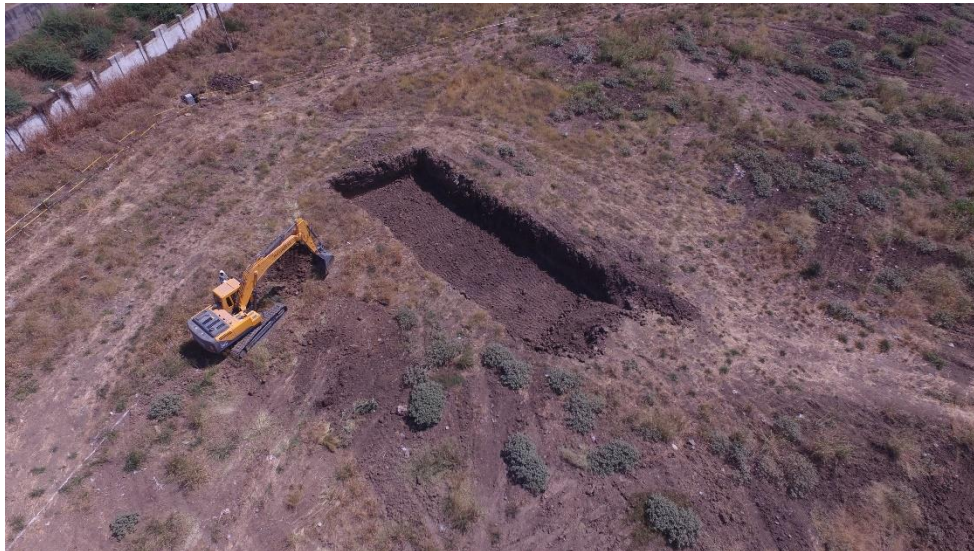
Water reservoir work
