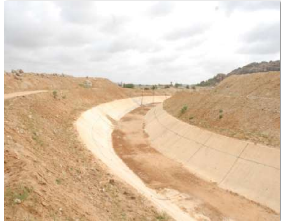
Irrigation Project in Telangana State
