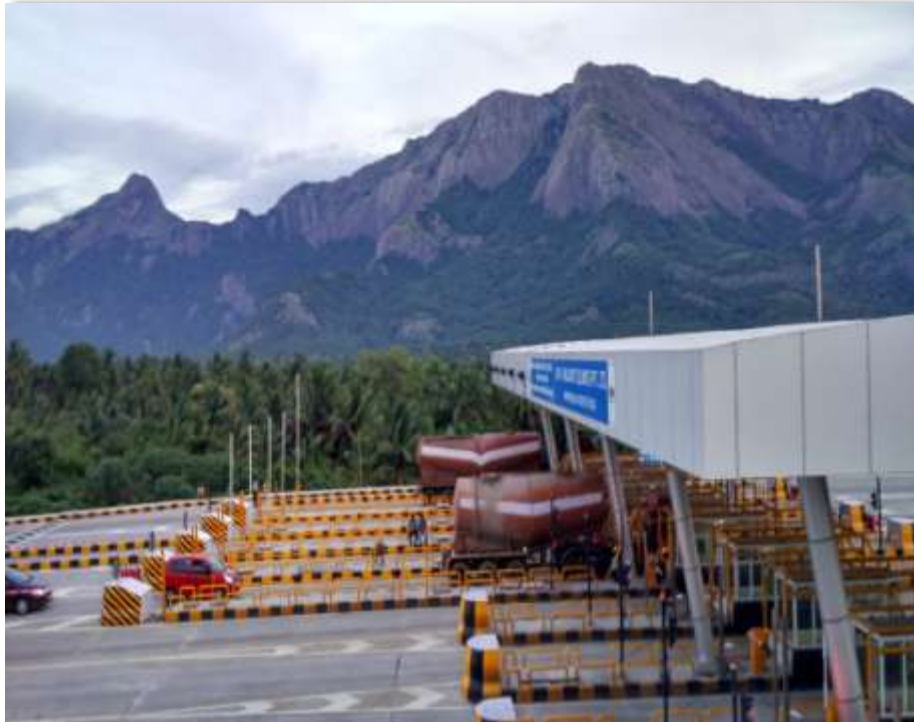
Walayar –Vadakkancherry BOT (Toll Road ) Project, Kerala
