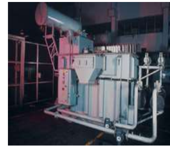
Furnace Transformers
