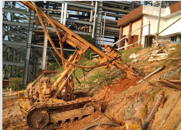
Drilling for Slope Stability at MRPL, Mangalore
