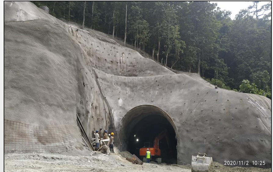
Railway Tunnel Project, Sikkim
