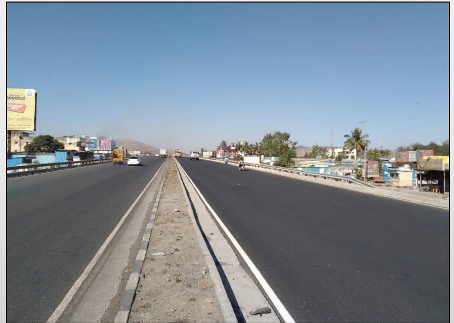
Pune Satara Road Project
