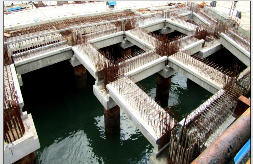
ANDAMAN LAKSHADWEEP HARBOUR WORKS, PORT BLAIR
