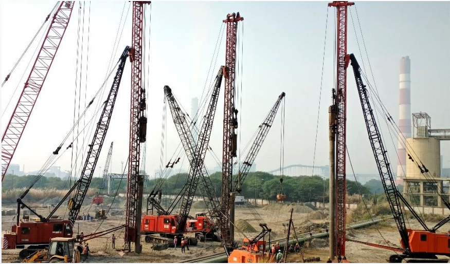
Stone Column & Piling Work at Power Plant, Anpara, UP
