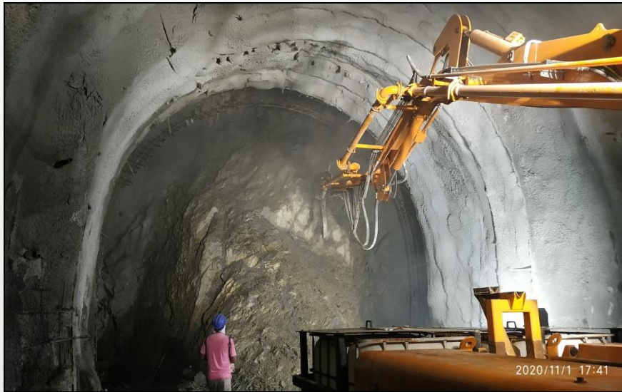
Railway Tunnel Project, Sikkim
