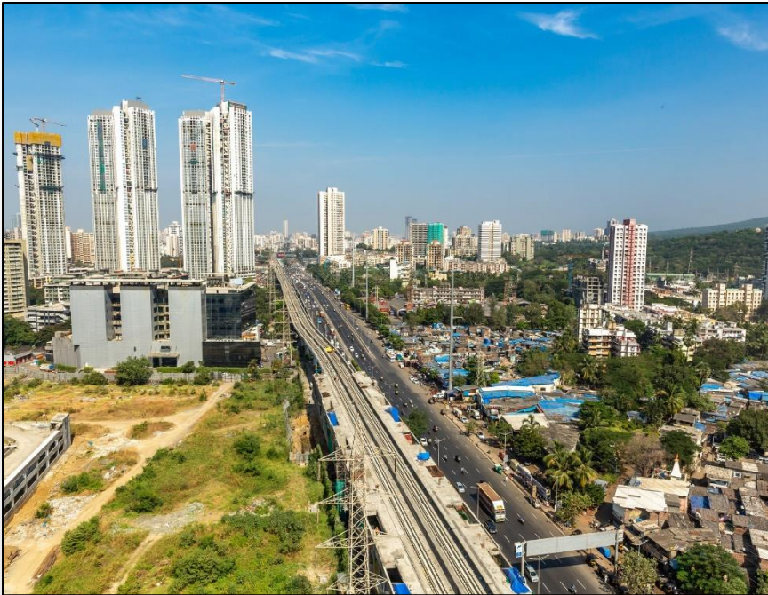
Track Work Line 7, MMRDA Mumbai Metro
