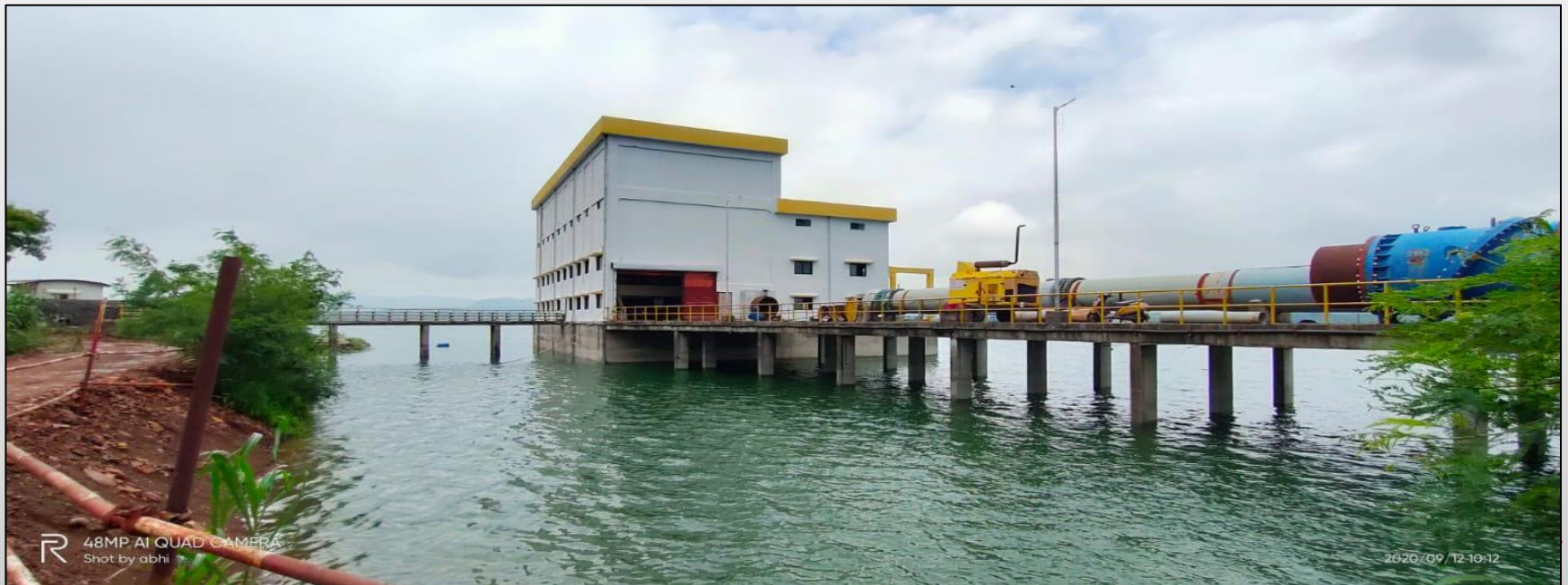
Bhama Water Project, Pune
