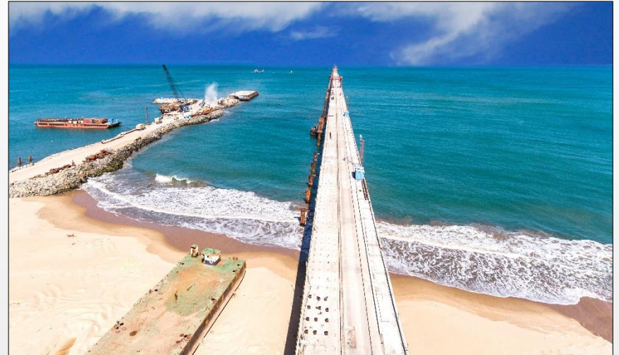
Udangudi TANGEDCO, Coal Jetty, Tamil Nadu
