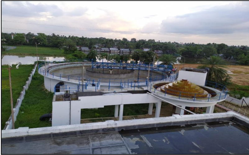
Aerial View of WTP at Rampur, Agartala
