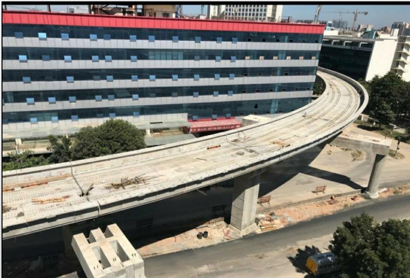
Bangalore Elevated Metro Project
