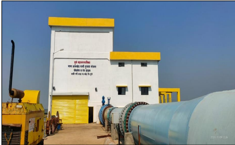
Intake Works at Bhama Askhed, Pune
