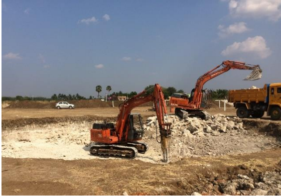
Site Installation underway
