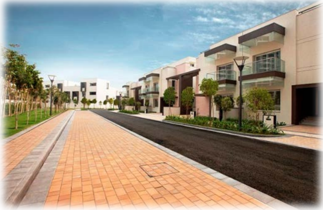
International City, Row Houses (Phase 1), Gurgaon
