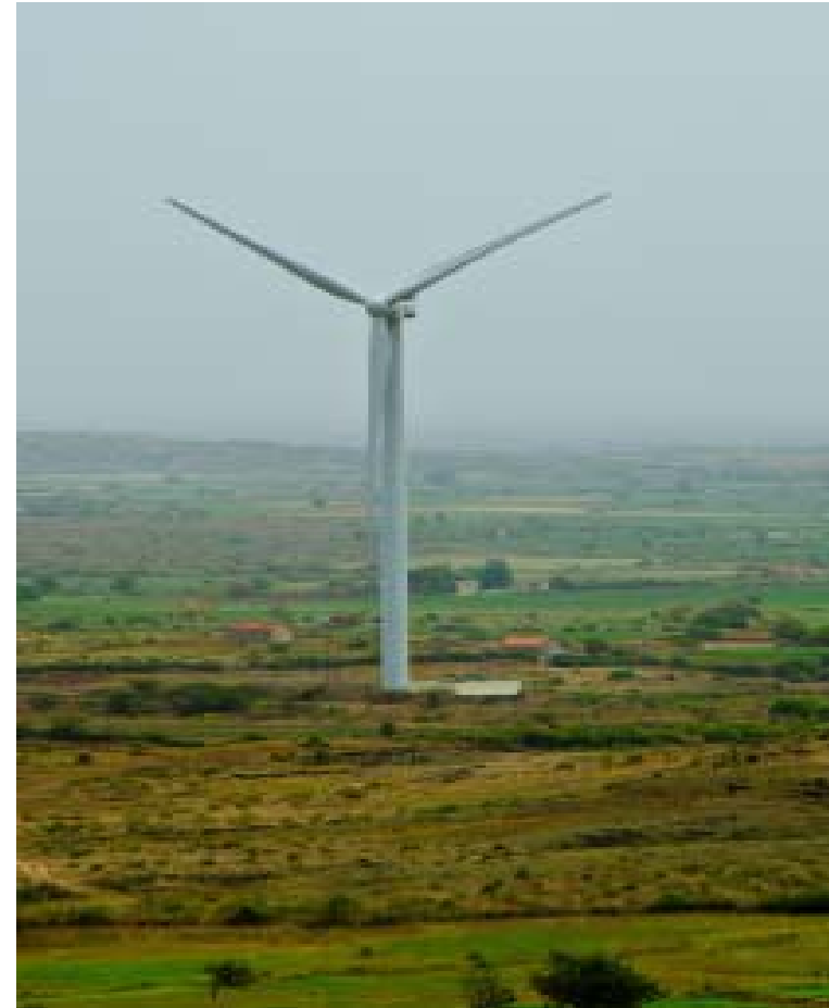
CESC wind sites in Jaisalmer, Rajasthan
