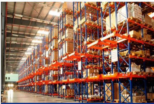
RACKING SYSTEM INSIDE ADC
