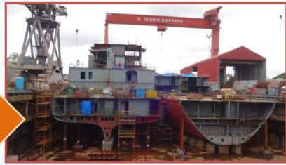
Commenced Block erection of 500 Pax cum 150 T Cargo vessels (2 nos) for A&N Administration on 28 April 2018. Project at advanced stages. Scheduled for launching by end Sep 2018.
