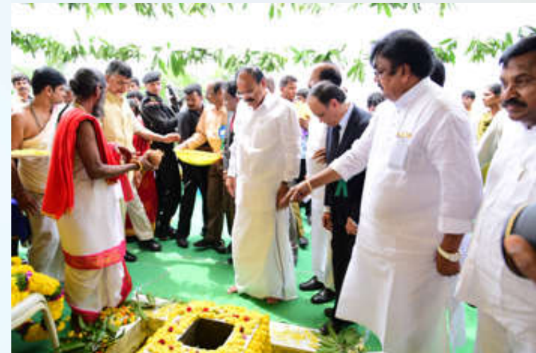
Laying the foundation stone for the Advanced Night Vision products factory at Nimmaluru, Andhra Pradesh
