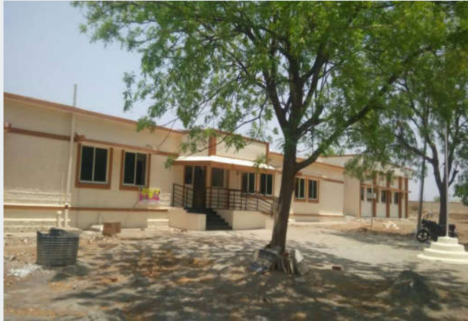
Construction of Wards, Mortuary Room, Toilets, renovation of existing OT and Labour room, providing ACs, Solar Lights, Furniture, DG set, Ambulance and medical equipment at Primary Health Centre, Mahagaon Cross, Gulbarga
