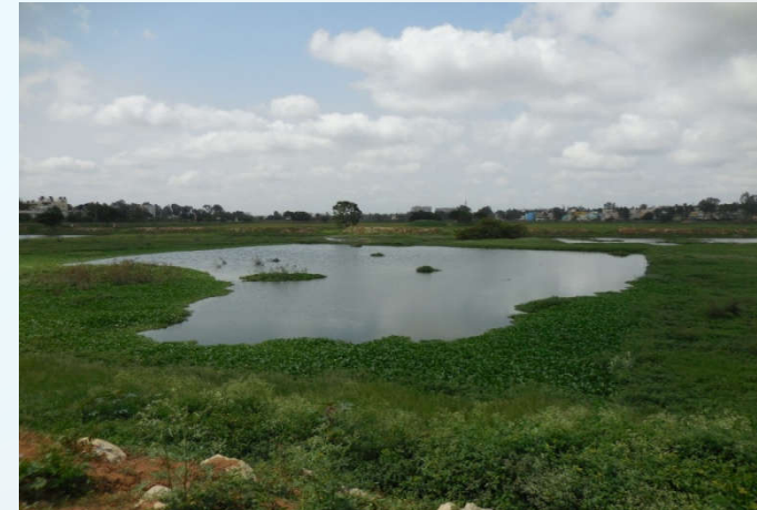
Supply, Installation & Commissioning of 10 MLD Sewage Treatment Plant at Doddabommasandra Lake, Bengaluru
