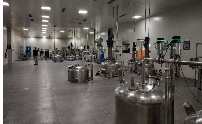
PLC Based touch less Manufacturing Set Up
