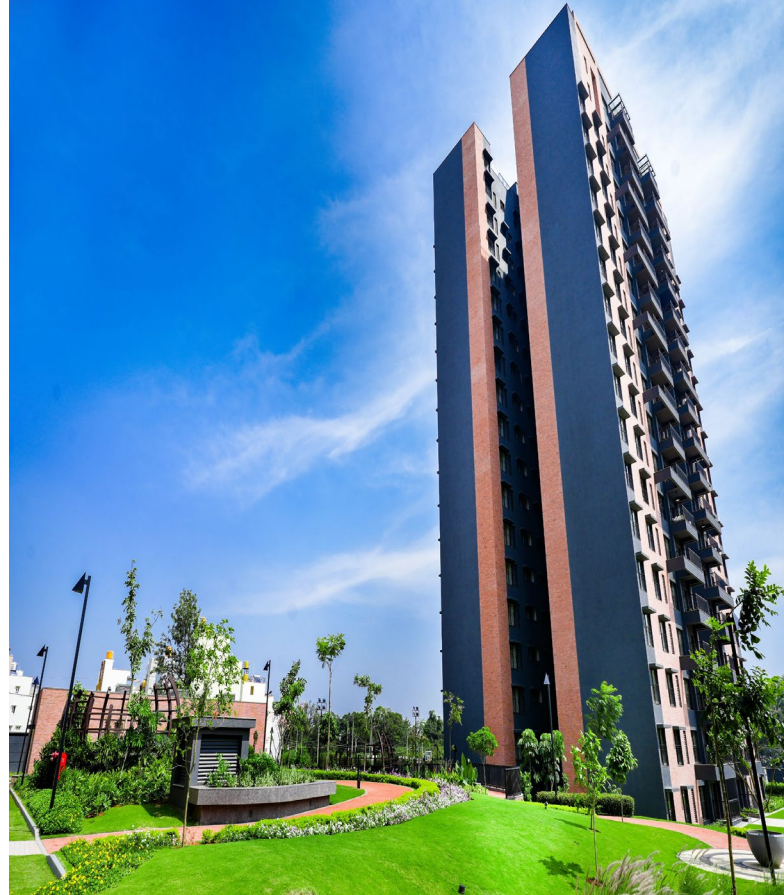
Wing 1 & 2 comprising of G+19 floors Total SBA completed in Q4-FY23 – 296,251 sft (155 Units)
