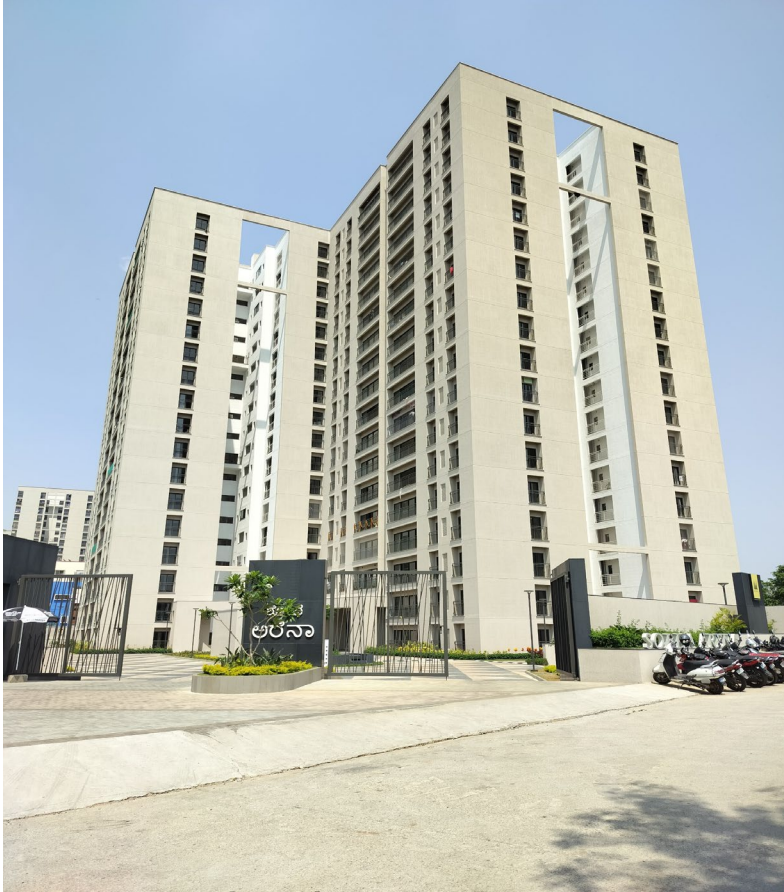
Wing 2 comprising 1 Tower of G+17 floors Total SBA completed in Q4-FY23 – 129,245 sft (68 Units)
