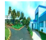
KSB MIL Controls Ltd. Meladoor, Kerala
