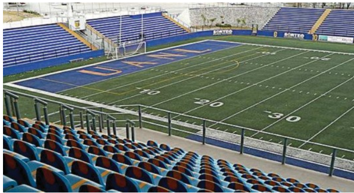
GASPER MASS STADIUM, MEXICO
