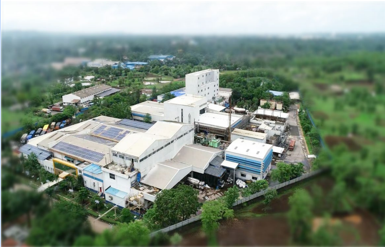
HUL's Dapada Home Care Factory
