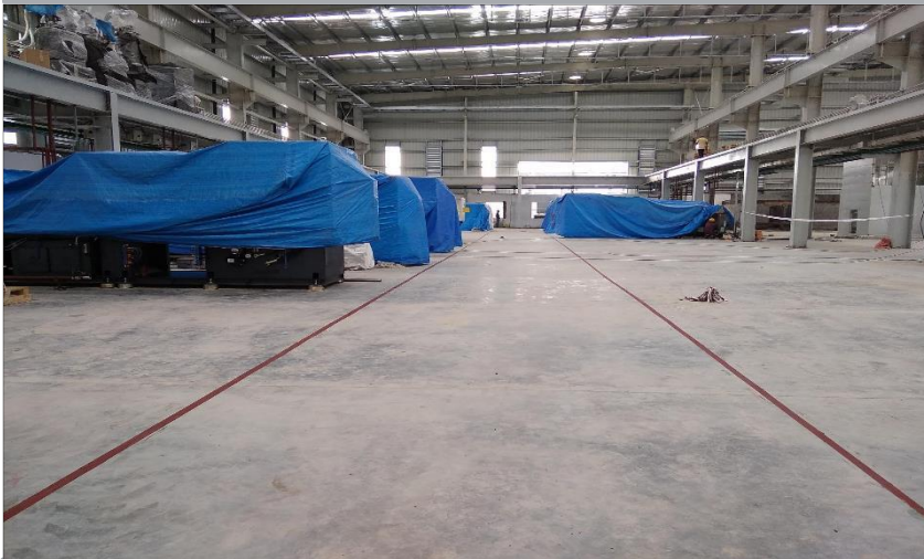
Surface treatment-hard coat installation
