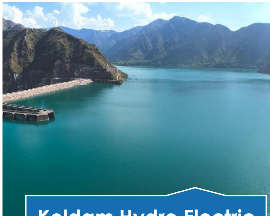
Koldam Hydro Electric Project
