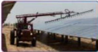
Innovation in Module Cleaning System (Semi - Automatic)
