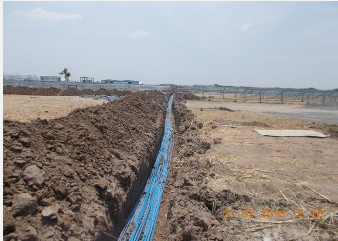
DC Cable Laying & Termination
